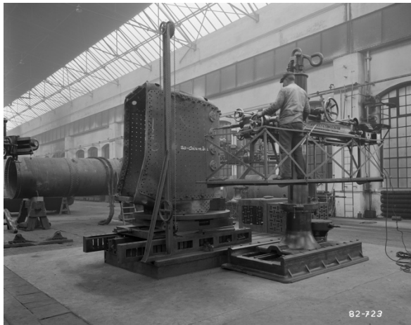
Fig. 2. Skoda workshops, Cutting threads for roof screws, 1928. [4]
