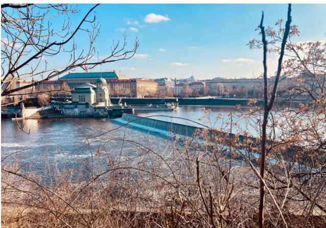
Fig. 4. Štvanice hydroelectric plant and Helmovský weir. [29].
